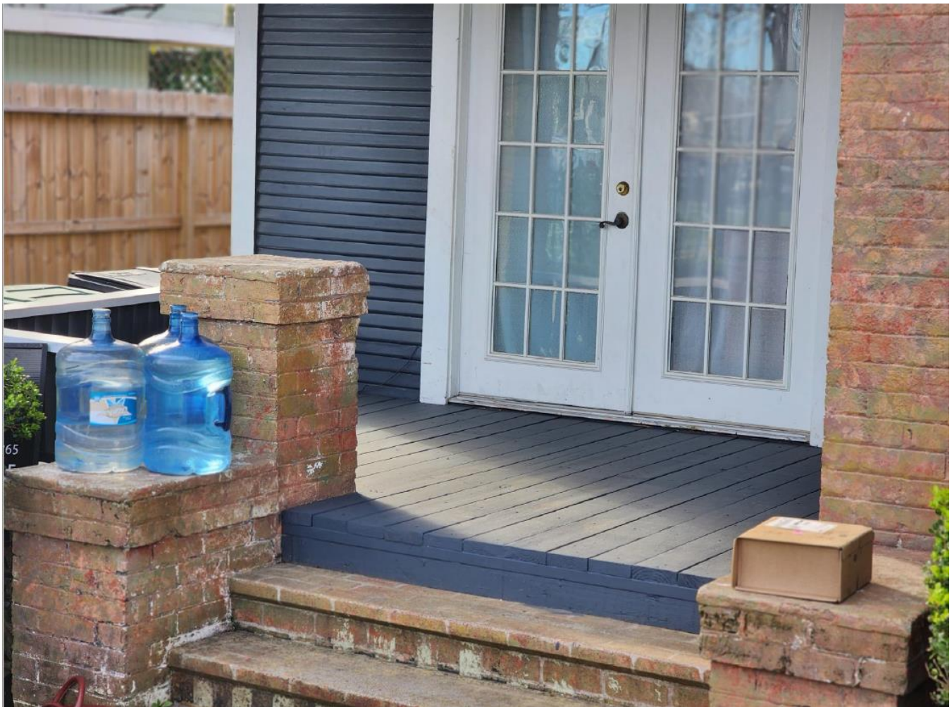
Figure 6 - Additional View Close Up of Deck
