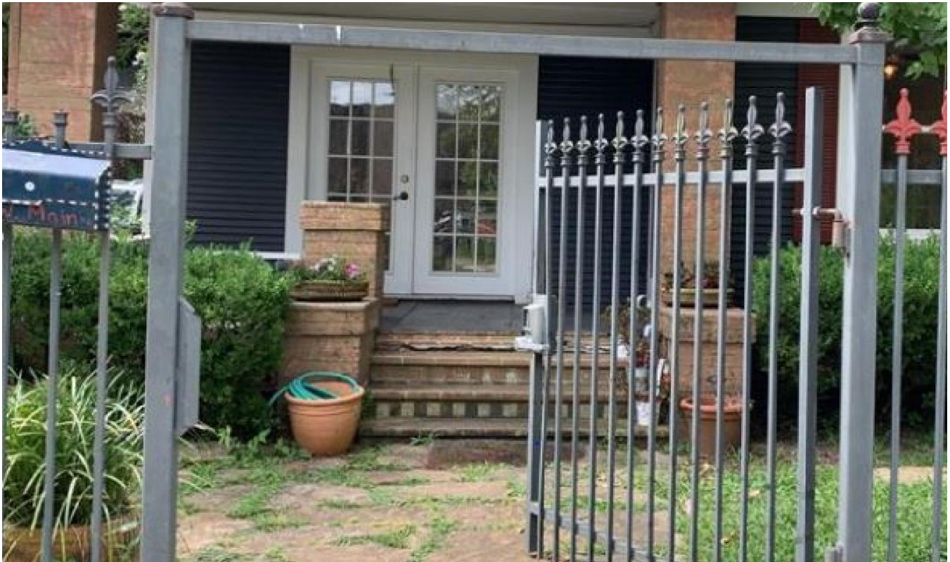
Figure 2 - View of Porch Floor Prior to Alteration from Google Streetview
