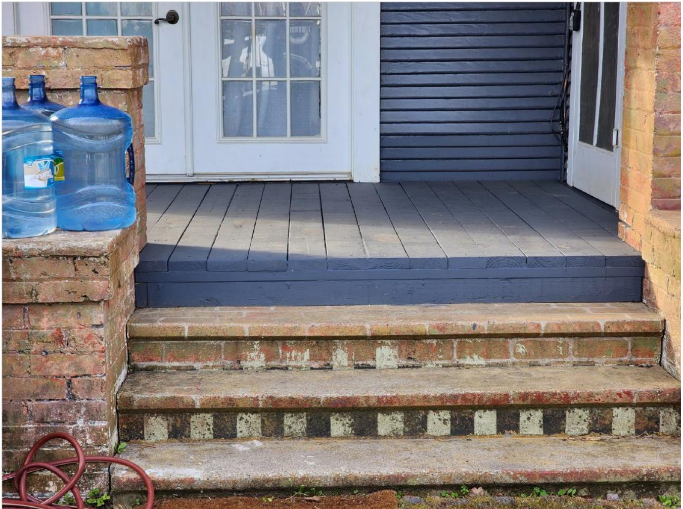
Figure 5 - Close up of new decking
