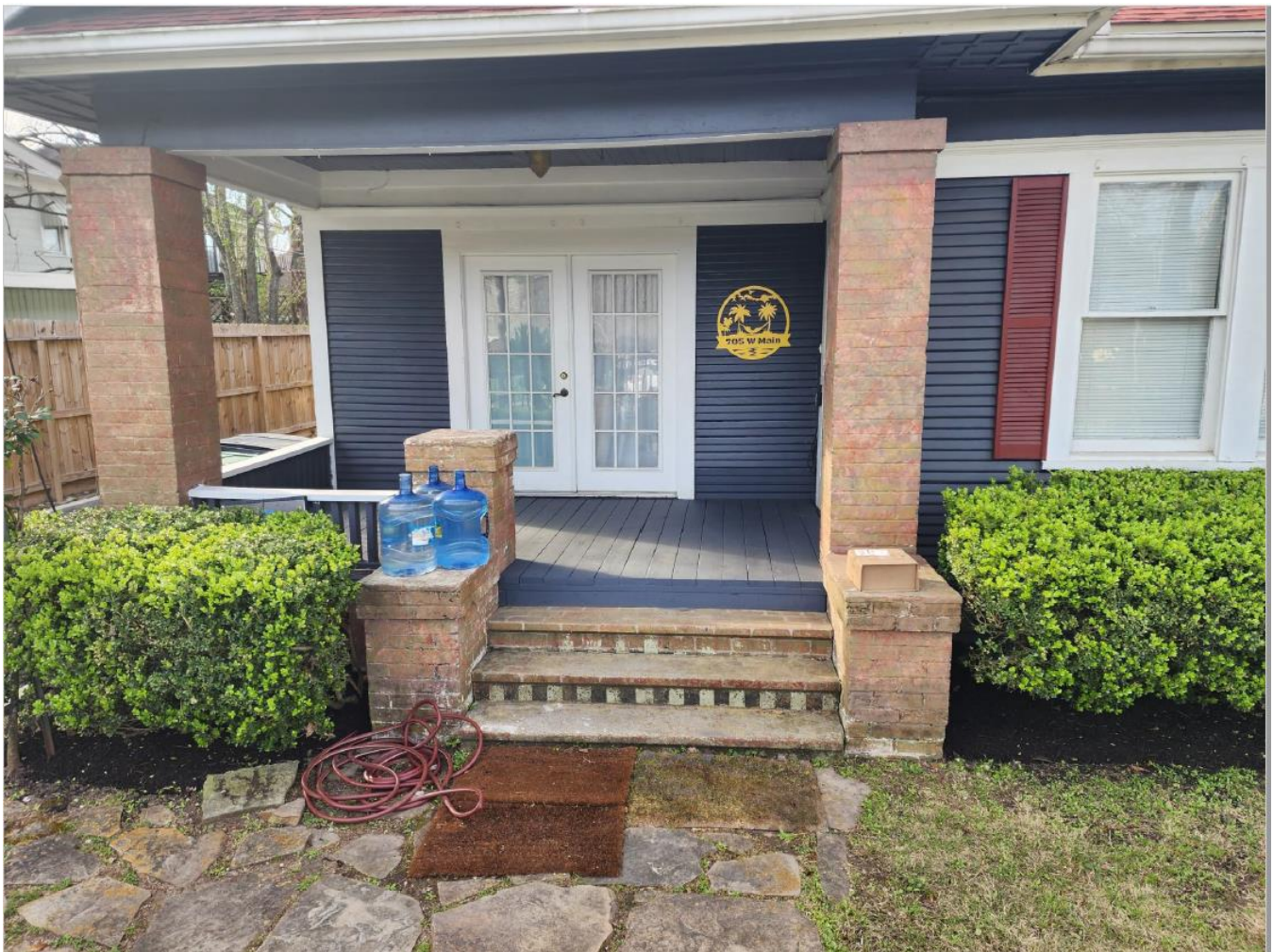
Figure 4 - View of porch floor after work completed
