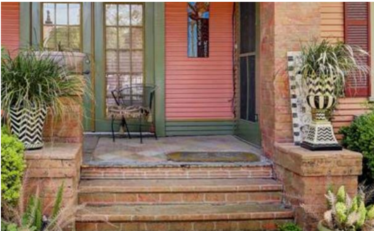
Figure 3 - Image from HAR Listing Porch Floor Prior
